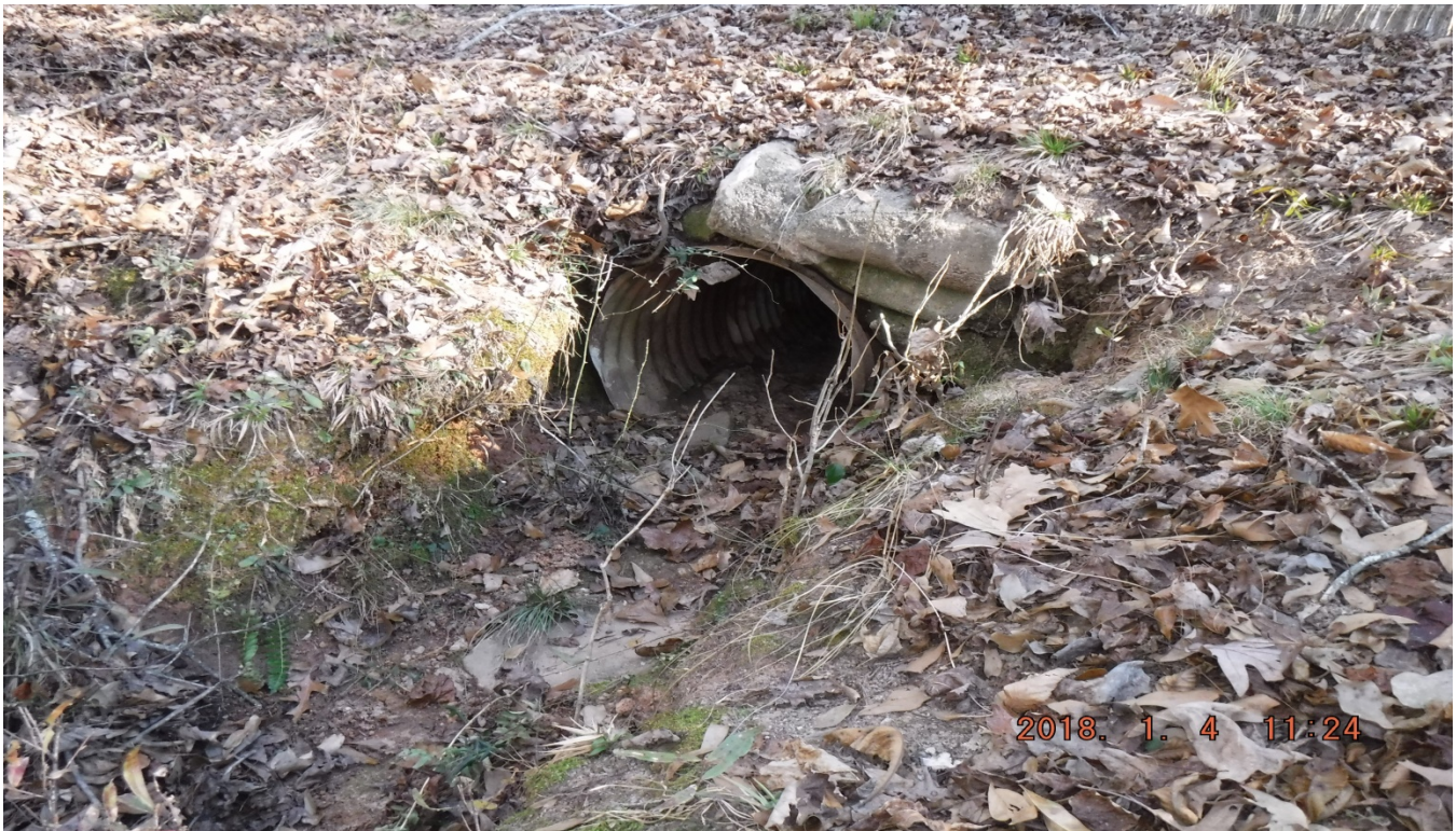
Photo 1: Pipe condition prior to replacement. (01/04/2018)
