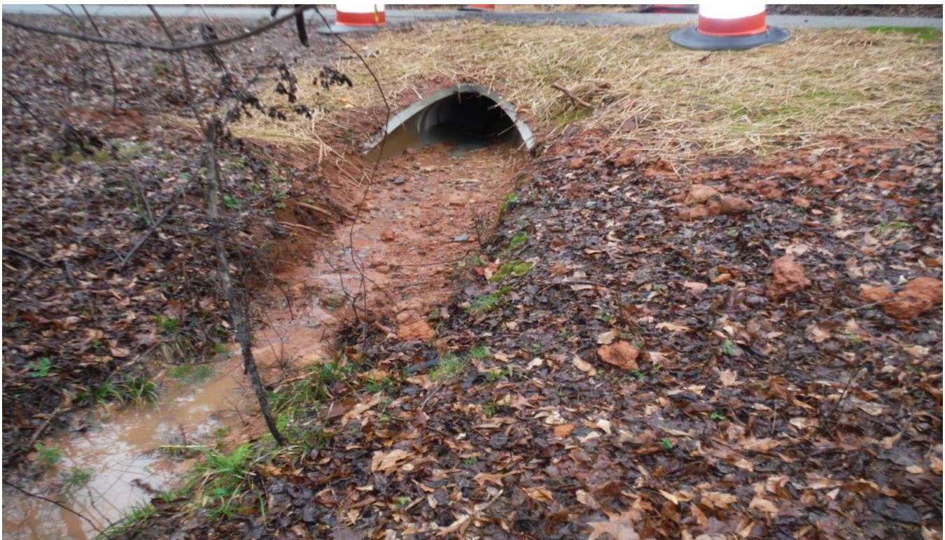
Photo 2: New pipe has been installed and soil stabilization placed along project location. The project was completed on 02/20/2018. (02/28/2018)
